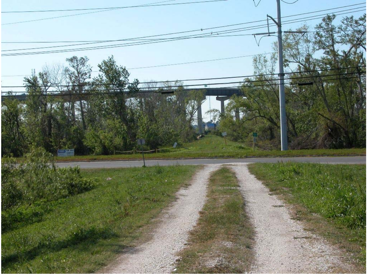
Back Levee intersects Hwy 406 looking toward the GIWW and General De Gaulle Bride overpass. No closure at Hwy
