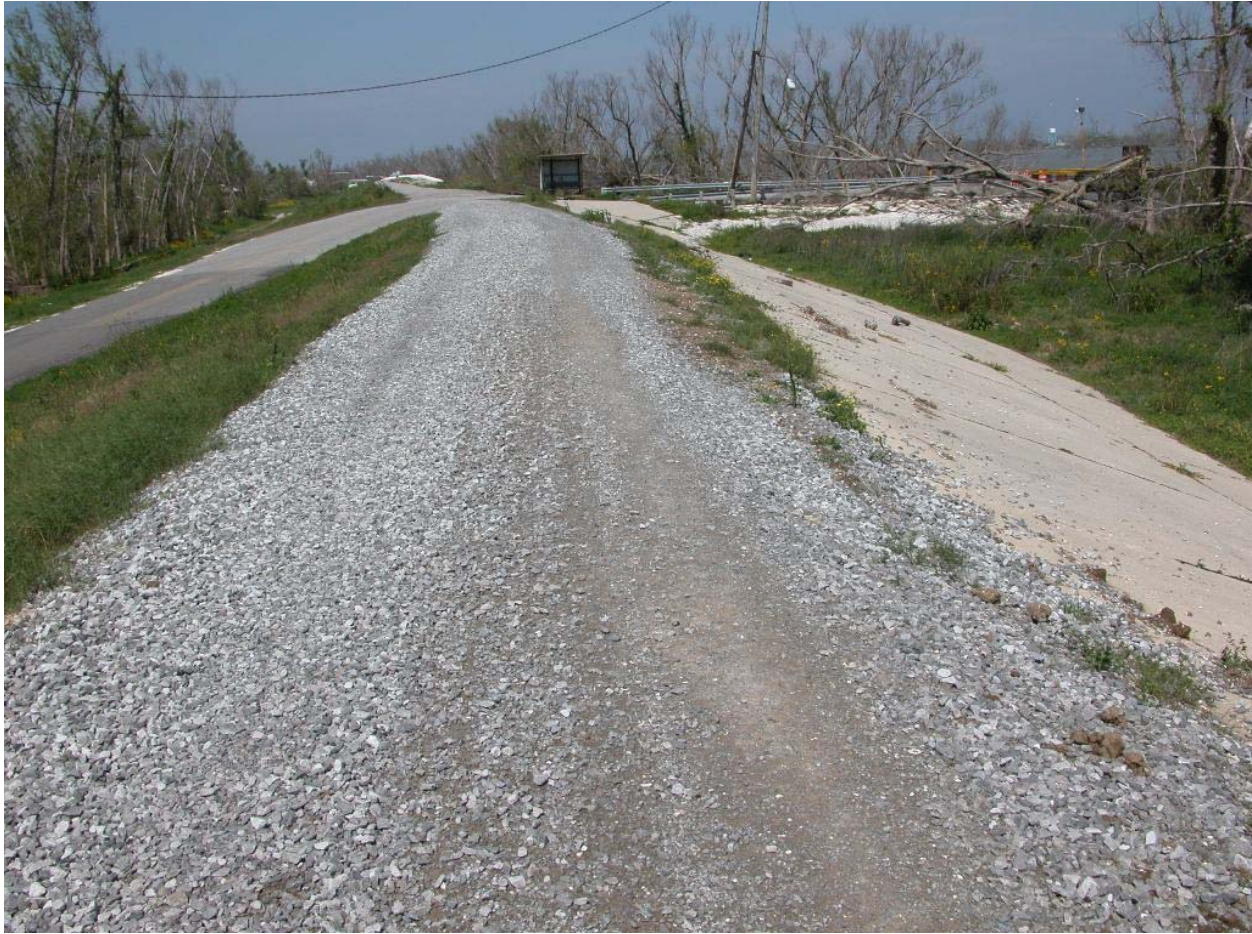
More typical condition along this section of the MRL, with concrete paved or stone crown and concrete armored floodside
