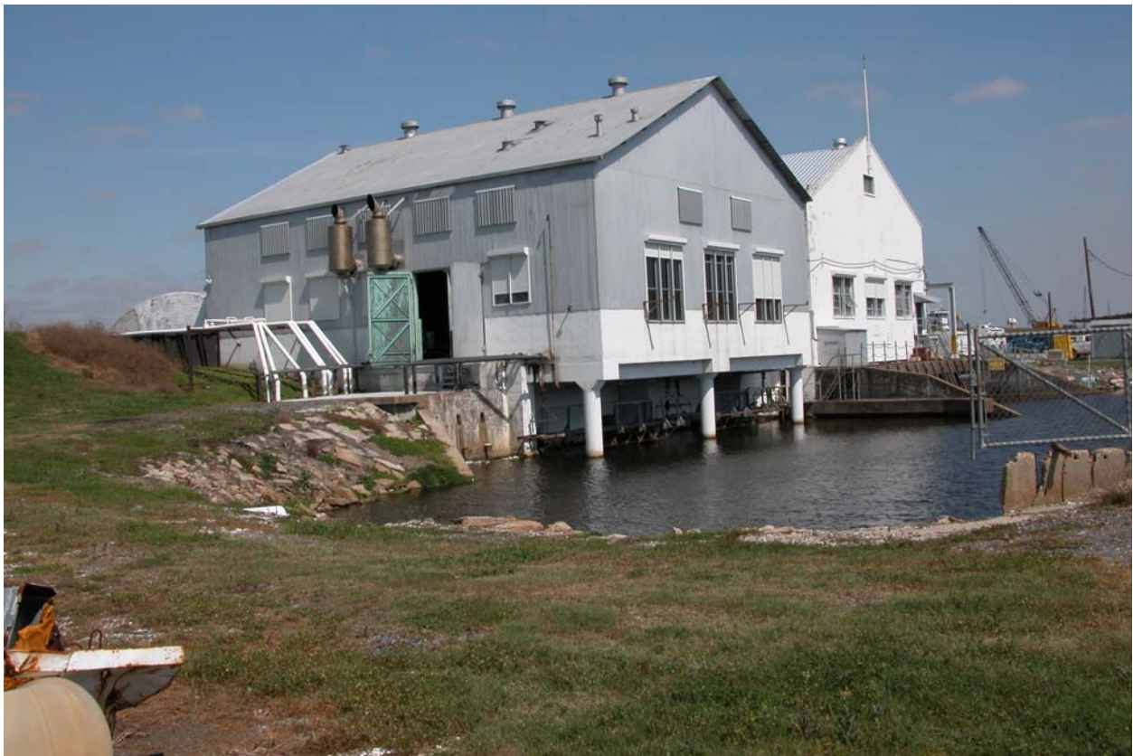
Plaquemines Pump Stations 1 and 2
