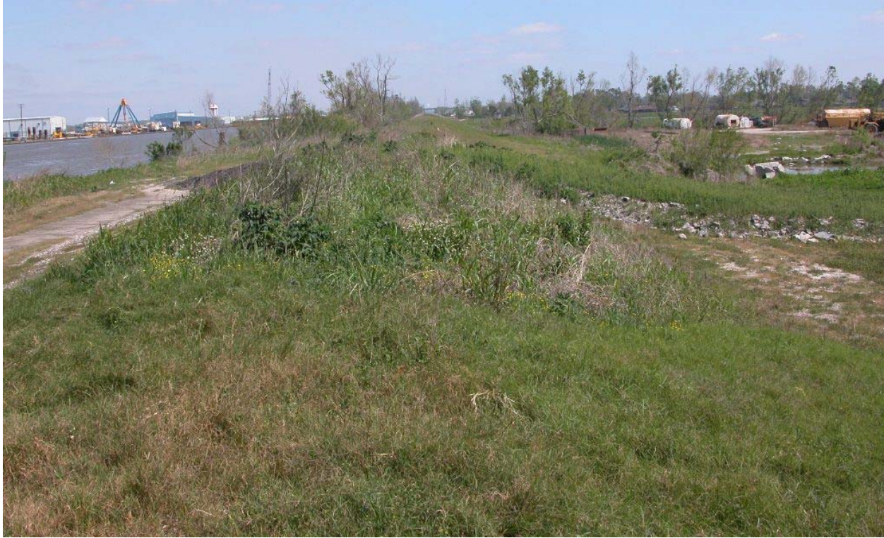
A point of levee erosion along the GIWW, however most is in good condition
